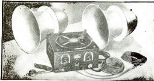
A 20-W., "beam"-type "campaign" sound system. (1188)
